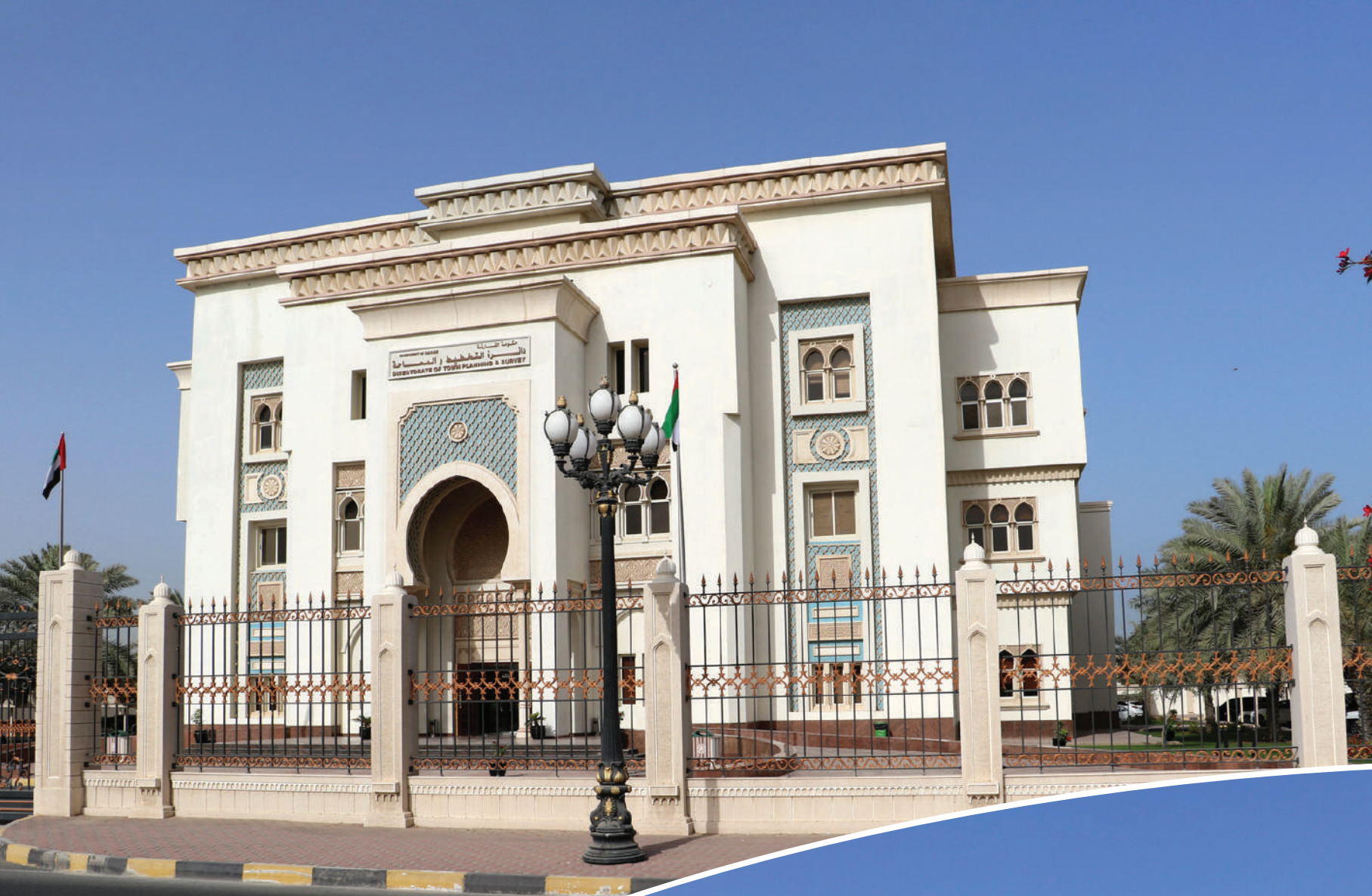
Department of Town Planning and Survey Building - Sharjah
